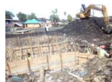
Site clearance and construction of a box culvert
