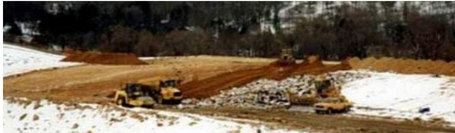
Figure 1. Application of daily cover
