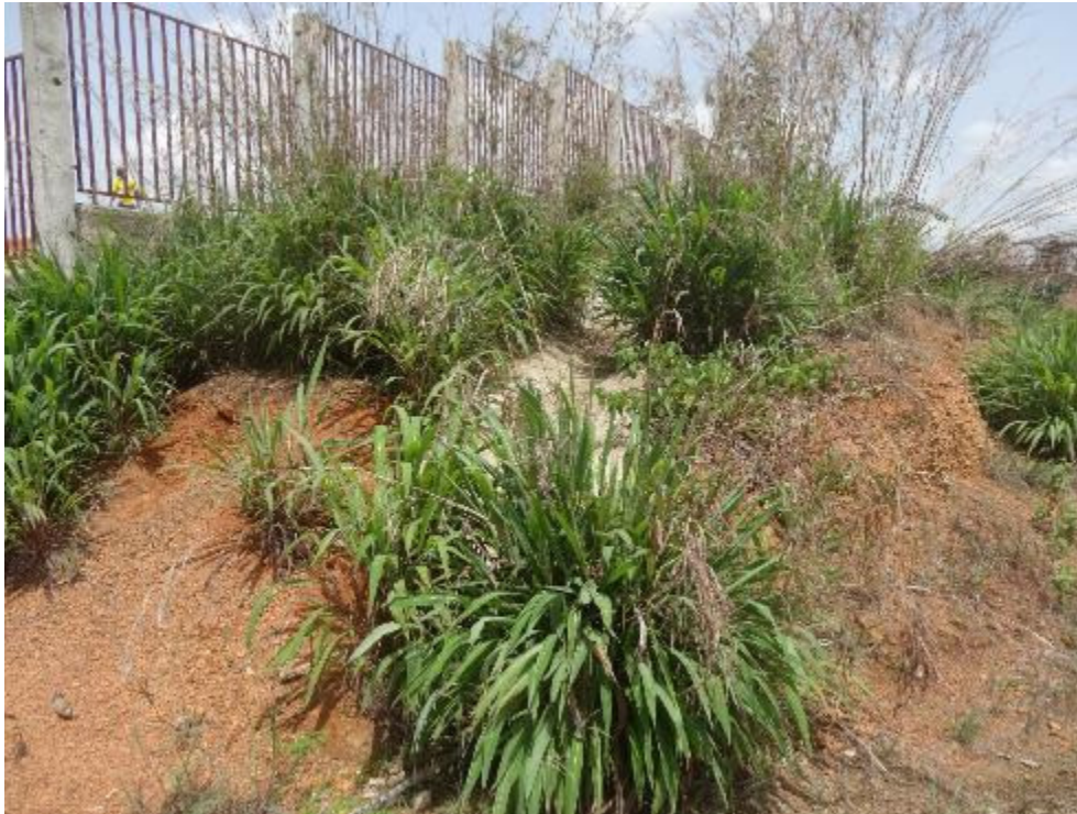
Overflow ducts from SALWACO site
