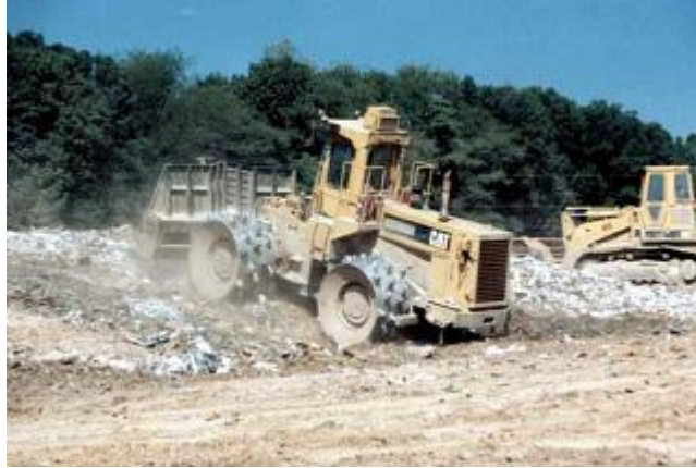
Figure 3. Wastes compacted by bulldozer/compactors
